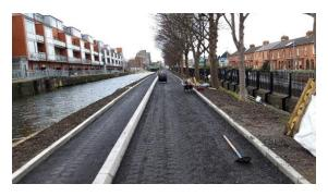
Kerbing installed on north side towpath between Cross Guns Bridge and Lock 4
